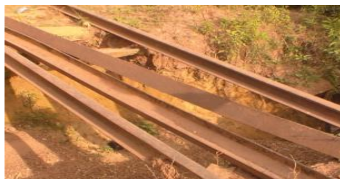
Figure 5.10 Closed Rail Line to Abura Undermined by Galamsey
