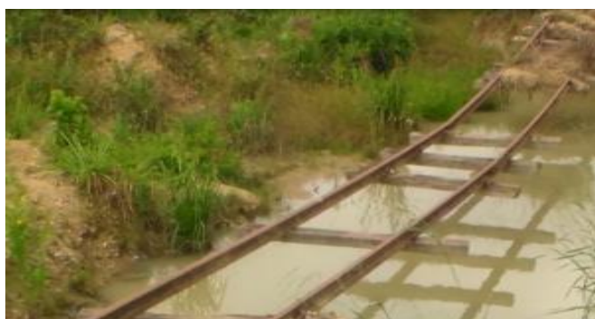
Figure 5.10 Closed Rail Line to Abura Undermined by Galamsey
